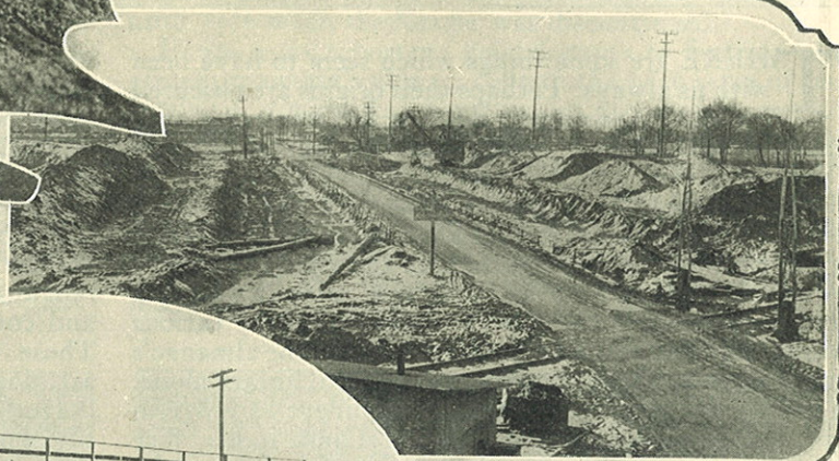
Above: Preliminary work for the extension of the yard over Leonard Avenue. There will be 30 yard-tracks bridged over this highway when the work is completed. Below: Members of the Engineering Department on the job at Columbus. Front row, left to right: J. P. Maloney, resident engineer; A. C. Tinsley, transitman; H. B. McColligan, transitman; L. G. Simmons, inspector; K. S. Pedigo, student chainman, and V. D. Johnson, resident engineer. Back row: C. H. Hughes, inspector; T. G. Mebs, chainman; W. R. Staples, inspector, and P. C. Turner, contractor
